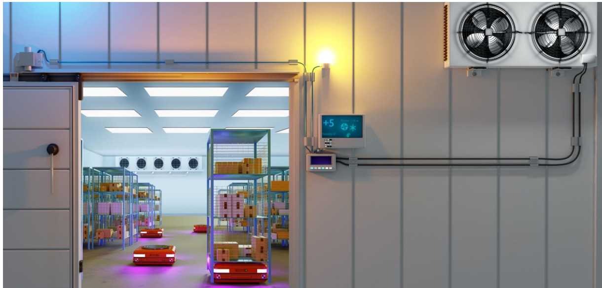
Figure 2. Vegetable storage automation warehouse
